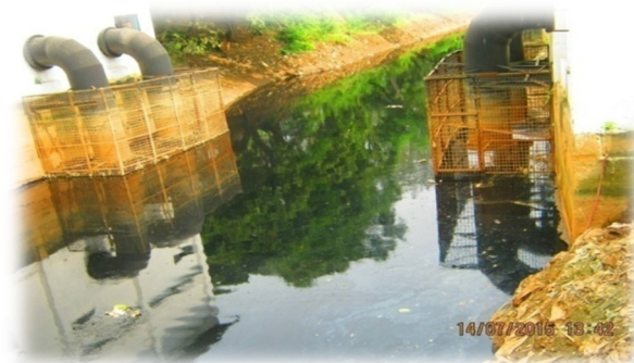
Drainage outlet at Bharalumukh
