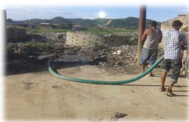
Untreated Leachate pumped out at Boragaon
