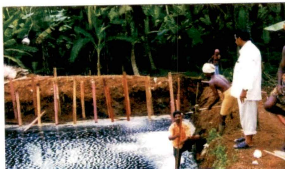
Leachate collected in temporary ponds
