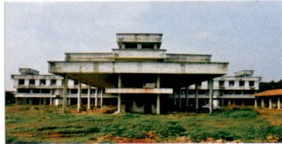
Bus terminal under construction
