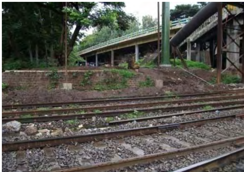
Ghorouri Yard. Pune open from all sides
