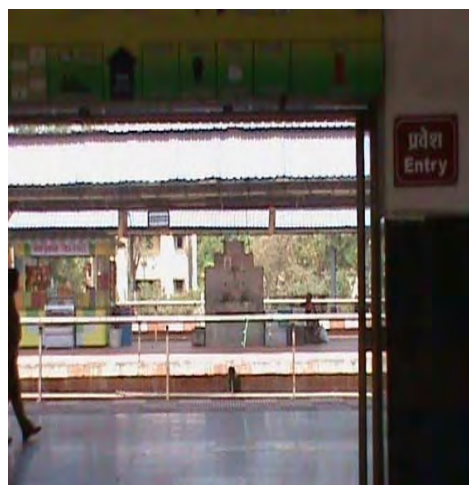
Unguarded entry to platform at Raipur station in SECR
