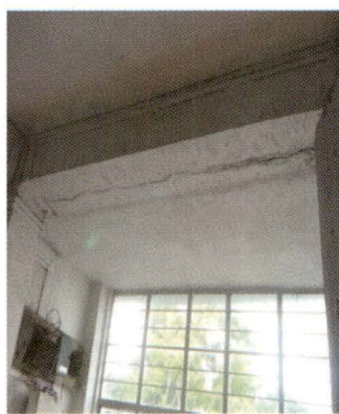
Cracks in a beam of Umsning CHC from where water seeps through.
