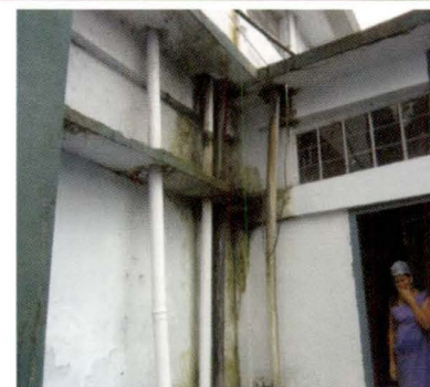
Leaking pipes and overflowing septic tank located next to kitchen area of Nongpoh DH
