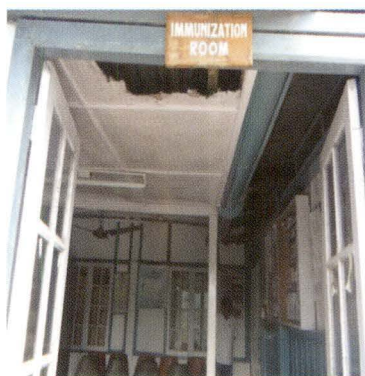
Hole in ceiling of immunisation room Umsning CHC from where rain water leaks
