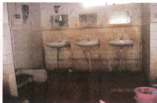
Toilets at boys' hostel No.7 & 8
