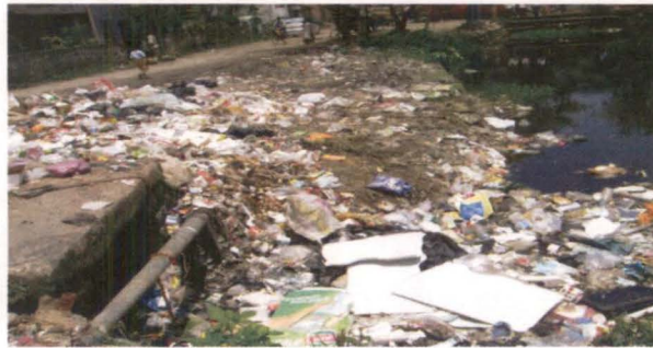
Storm water drainage at Jorhat (Toklaijan) (23 May 2010)
