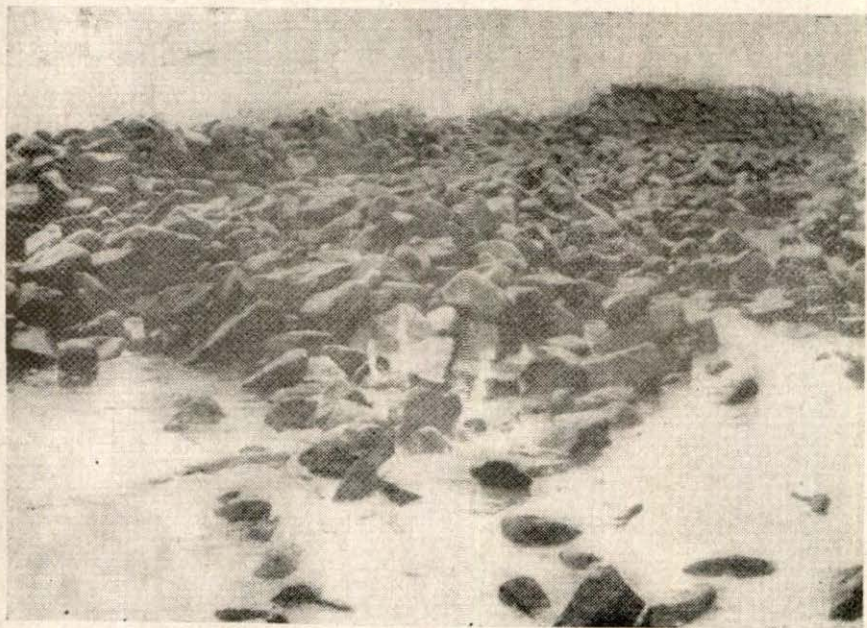
SUNKEN PORTION OF AN OLD SEA WALL WITH SCATTERED STONES REDUCED TO PEBBLE SIZE
