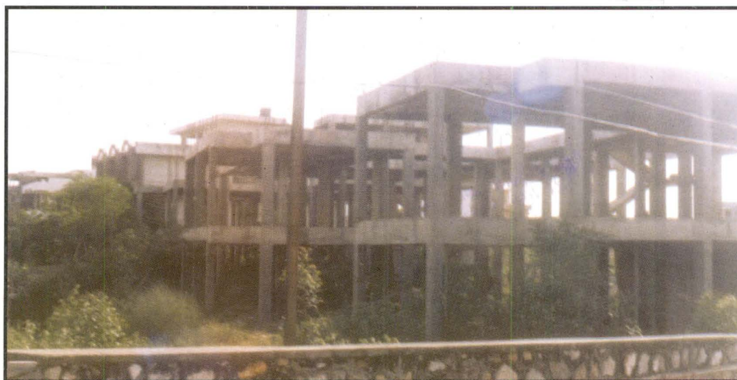
A view of incomplete staff quarters
