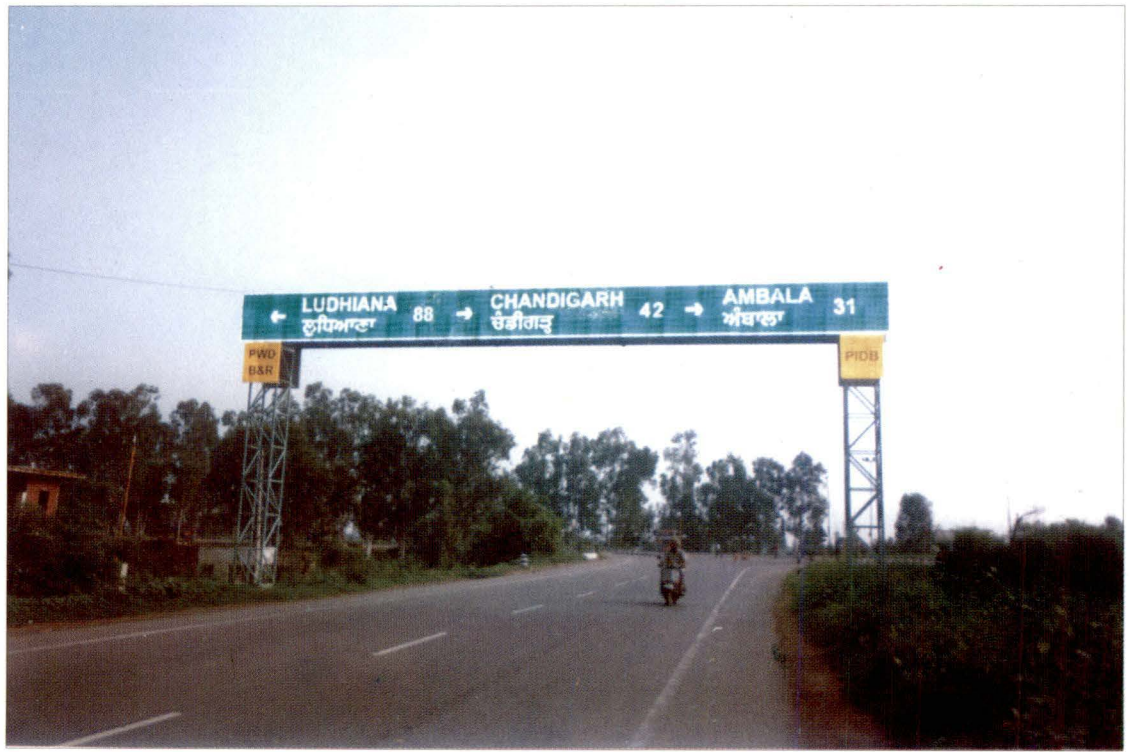
Photograph showing National Highway-64 upgraded out of PIDB funds by State Government (Refer paragraph 3.1.8)
