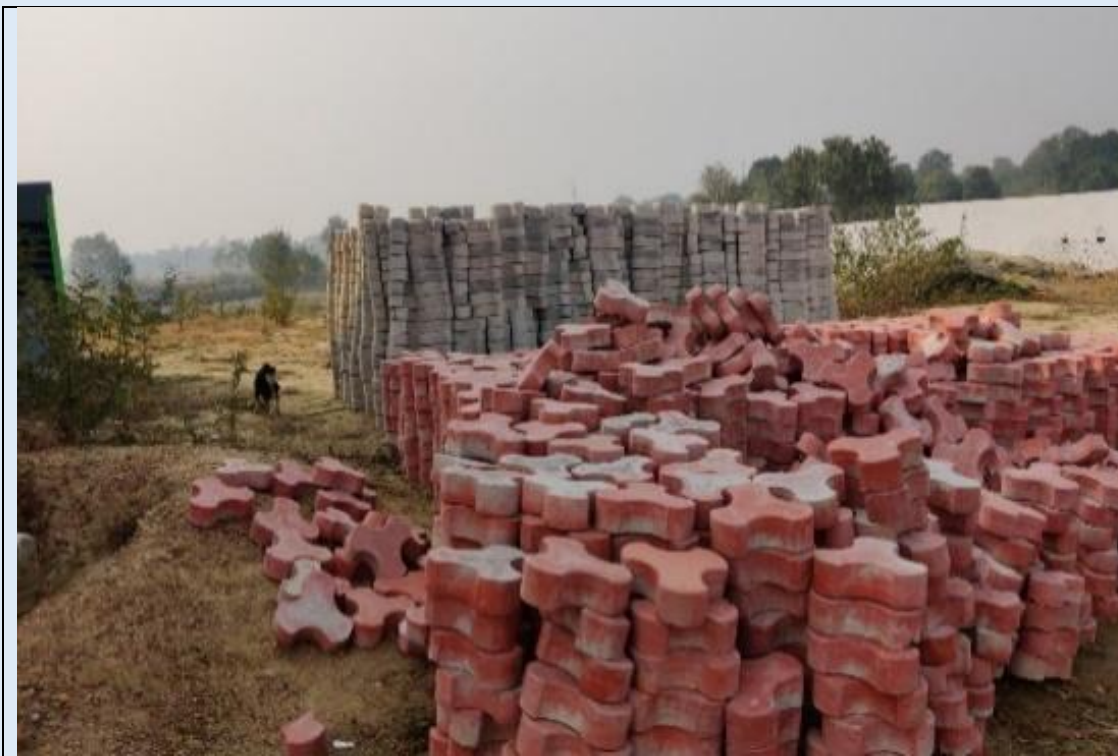
Picture 5.1: Construction of Paver Block under progress at Rain Shelter, Suiya, Bihar, which was however shown as completed in monthly progress report
