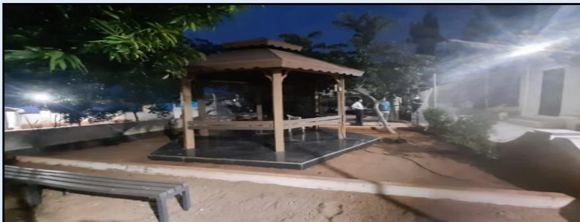
Picture 4.11: Gazebo constructed at Mulugu District Collector's Camp office in place of Gattamma, Mulugu, Telangana
