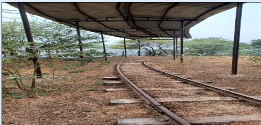
Picture 4.10: Outdoor shade structure erected in place of Maintenance Depot
