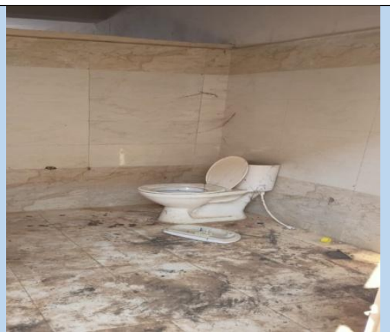
Picture 4.15: Sanitary fittings broken in the toilets provided at amphitheatre at Medaram, Tribal circuit, Telangana
