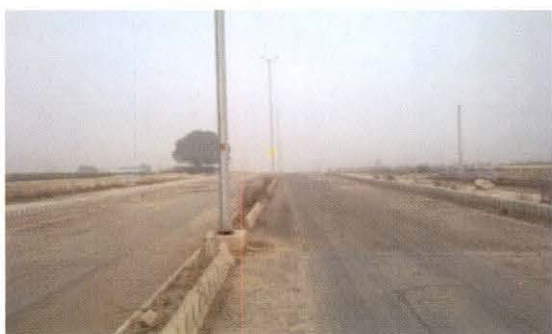
Rohini Zone: Construction of Main carriageway
