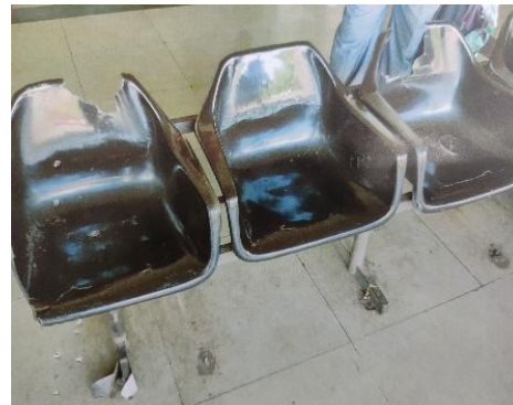
Picture No. 6.3.12: Damaged seats at Dharmasthala bus station (May 2019).
