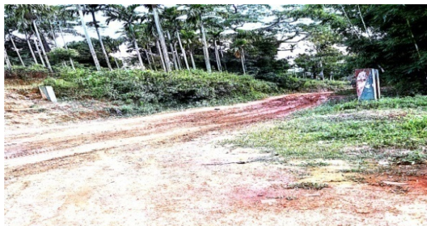
Photograph 2.2.1.: Poor road towards Nokrek.
