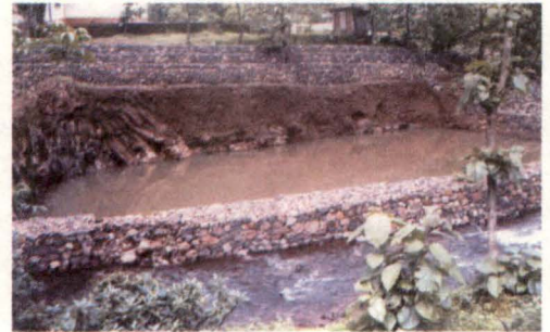
Water tank at Lanja, District Ratnagiri showing muddy water unfit for drinking.
