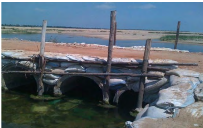
(Photograph of long path laid at Mudivarthipalem)
