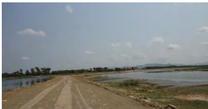
(Photograph of obstructing pathway at Chevitikallu sand reach)
