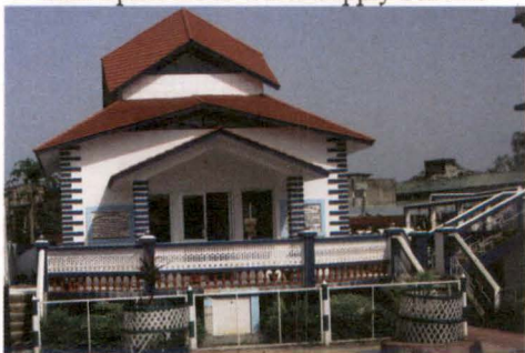
Ghungoor Water Supply Scheme
