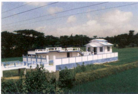
Srikona Part-II Water Supply Scheme
