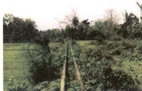
Lined canal of Udharbond ELIS, (Inoperative)/27 April 2010
