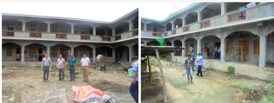
Front view of incomplete Boys hostel
