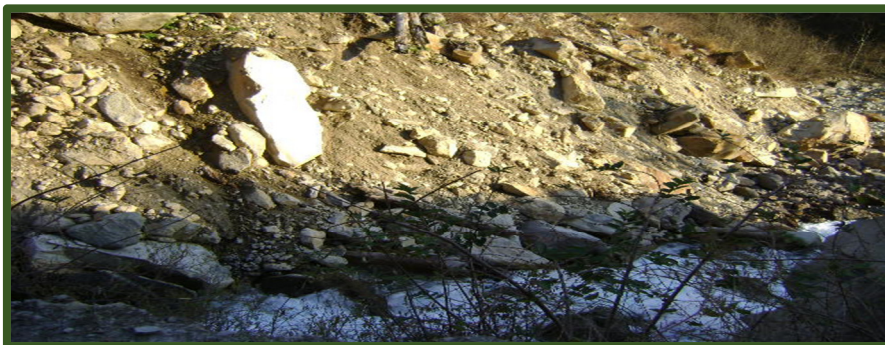
Ecological damage in the Sainj Hydroelectric project area Kullu, Himachal Pradesh due to non-treatment of Catchment Area
