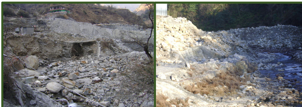
Muck overflowing to the river due to damaged muck site in Sainj Hydroelectric Power Project, Kullu, Himachal Pradesh
