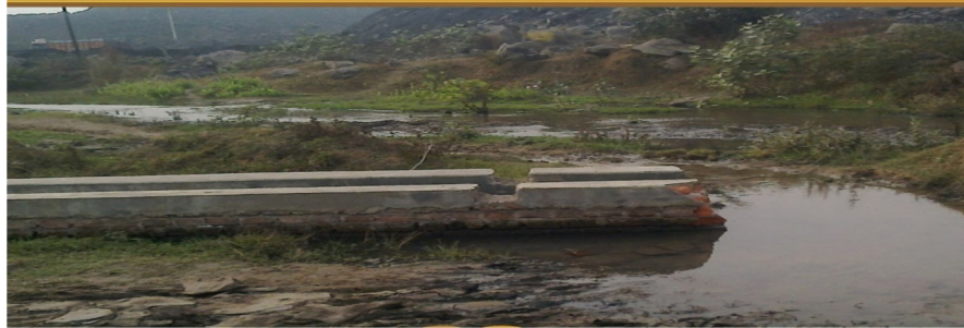
Water discharge in open area at Mohanpur OCP, West Bengal
