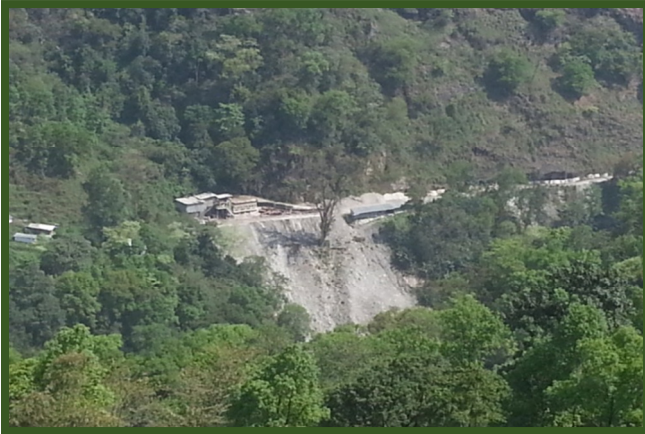
Dumping site at Lingdok, Sikkim
