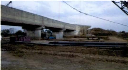
Repair work of aqueduct on Upper Stream side under progress
