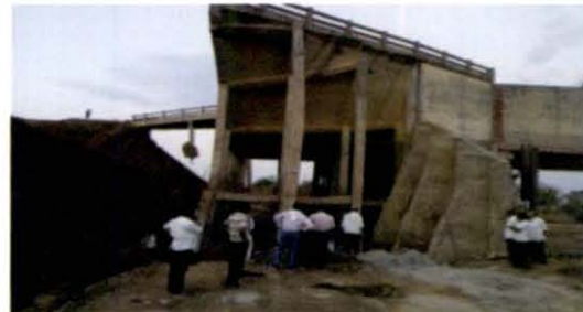
Repair work of aqueduct on Down Stream side under progress
