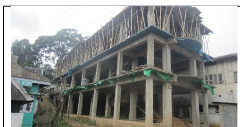
Photograph showing stage of completion of Court complex at Tuensang
