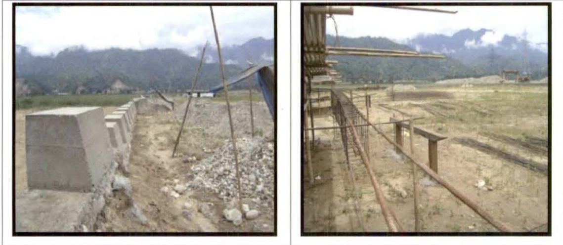
Construction of Inter State Truck Terminal at Lekhi (UIG)
