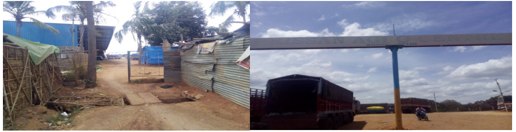
Photograph 2.2.3: Photos taken during joint inspection by Audit and Department staff on 26.6.18 show the entrance to Private Market through mandi wall and main entry from the road.
