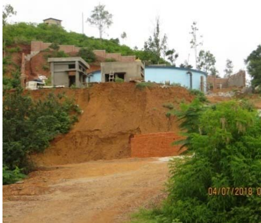
Photograph 3.1. Multi village water supply scheme works at Binkadakatti, Gadag Division
