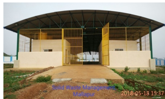
Photograph 2.2.7: Idle SWM Unit at Mallapur in Shivamogga district.
