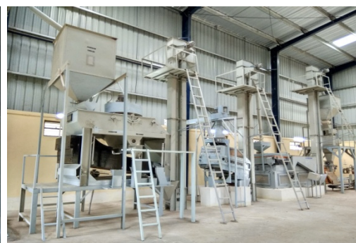
Photograph 2.2.2: Cleaning and Grading unit in Gajendragad, Gadag District which was completed during November 2016.
