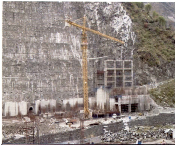
Back hill slope stabilization of power house of Parbati-II
