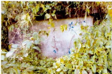
Non-maintenance of sedimentation tank at Bojogari
