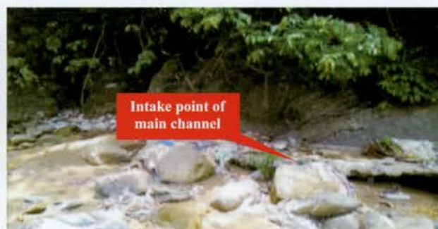
Channel without proper headwork at Fuanlui
