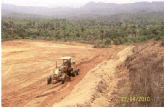
Talamba dam seat
