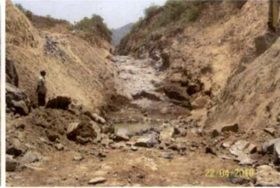
Talamba –COT work in progress
