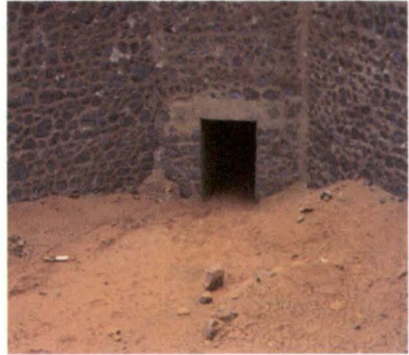
Tangar (main outlet at sill level)
