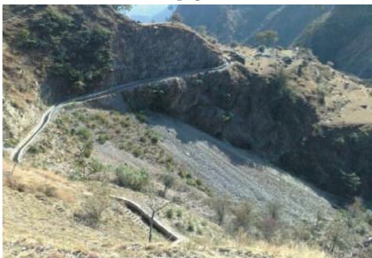
Uncovered hydel channel: Hydro Power Project Manjhal, Chamba District (Photograph dated 10 April 2012)
