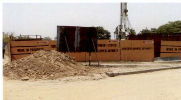
Construction of flyover next to the Games Village
