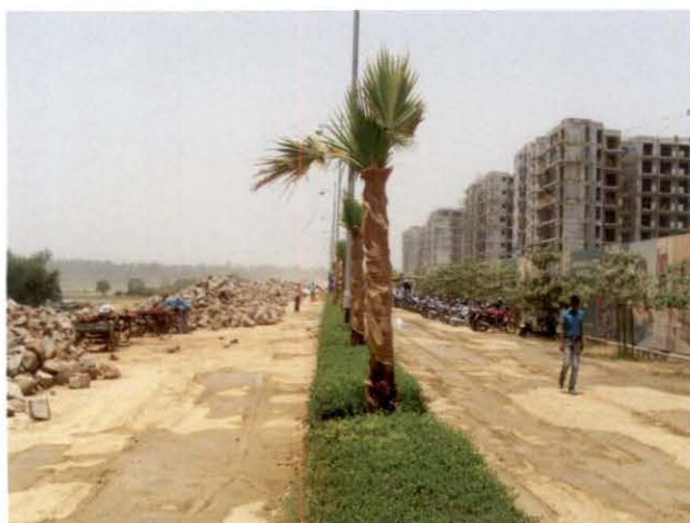
Construction of access road for players' entry in progress
