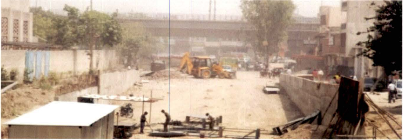
Construction at Vivek Vihar Flyover
