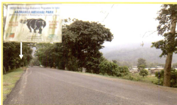
The signage of animal corridor on left side of NH 37 and the settlement of Deosur Chang on the right
