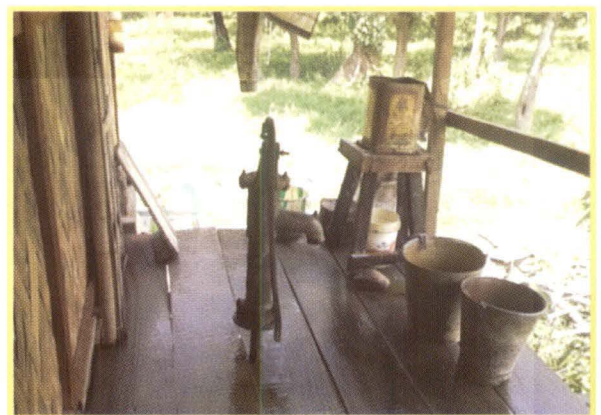
Hand pumps are installed in the camps - strategically elevated so that guards don't have to come down
