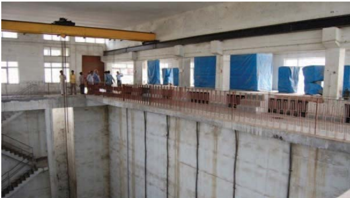
Incomplete Intermediate Pumping Station at Munsipurwa, Kanpur
