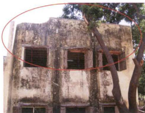
Broken parapet and sunshades in GPS, Muthirapalayam
