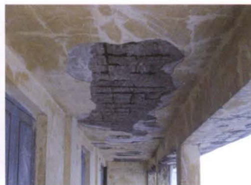
Damaged ceiling of verandha GHSS, Sultanpet
