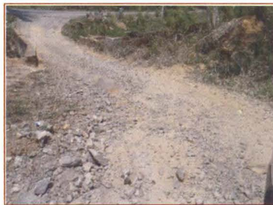
Picture 4.8: Bad condition of Kamarajar Road
