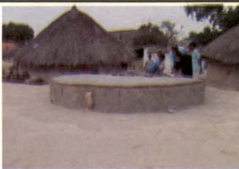
Structure of water tanka without roof attachment Bhanpura Village, Barmer
