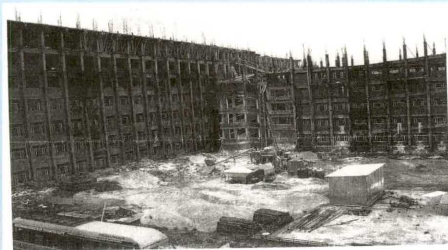
Photo: Work in progress of college building at Udaipur, Rajasthan (July 2008)
