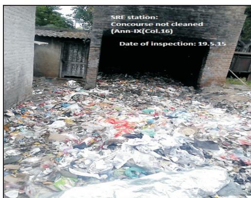
Garbage accumulation in concourse at Saharanpur station of A category (NR).
