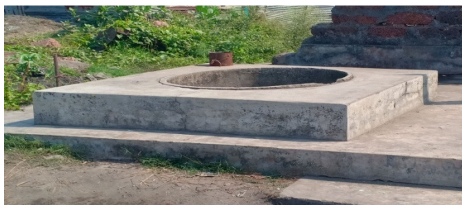
Dug well constructed without permission of CGWA
