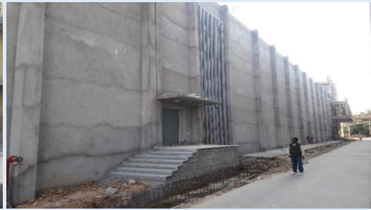
Rainwater harvesting structure
