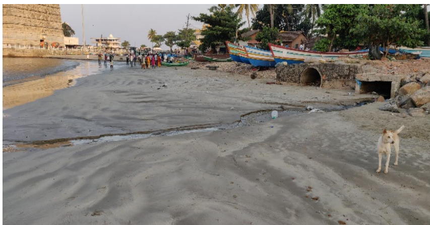
Fig. 30: Urban sewage directly entering coastal waters at Murudeshwar Beach
