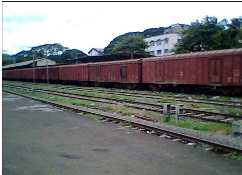
Partly covered shed at Pune goods shed
