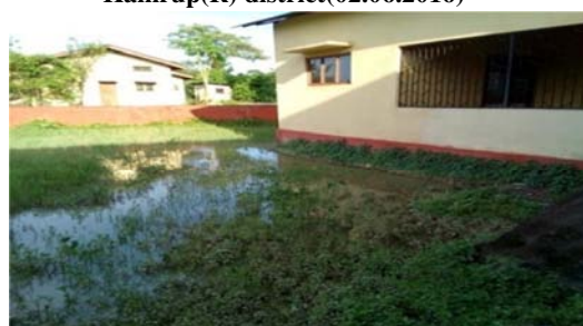
Water logging in Dakhinhengera PHC, Golaghat district (30.07.2016)
