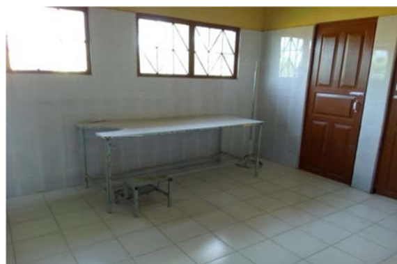
Labour room at Dakhinhengera PHC, Golaghat district remained non-functional due to want of trained staff (30.07.2016)
