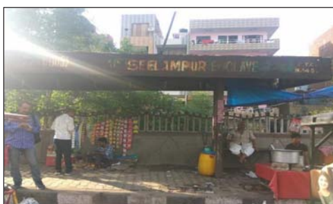
Figure 13 :Old BQSS with no seating space
