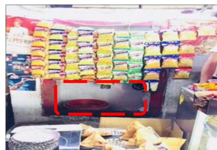
Figure 5: Fire Hydrants blocked by Kiosks
