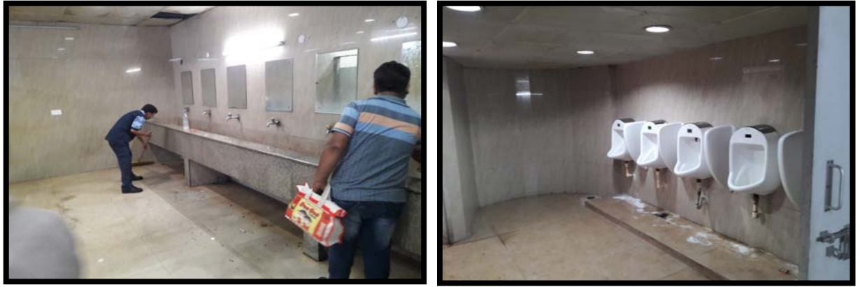
Figure 12: Kashmere Gate ISBT
