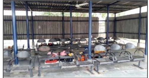
Figure 9: Broken chairs at waiting hall in SKK ISBT
