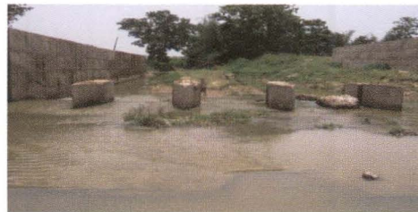
Laboc Flow Irrigation Scheme (4 June 2013)
