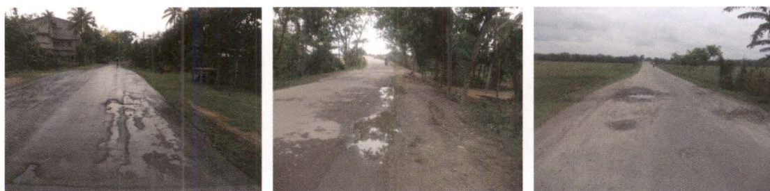
Improvement of Na-ali Ch 10 th km (15 May 2013)
