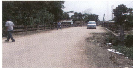
Approach Road to RCC Bridge on Silapathar Jonai Link Road (4 June 2013)
