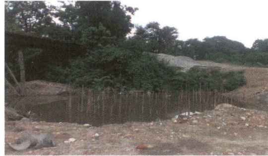
Bridge No. 32/2 on Dhubri Kachugaon Road (13 June 2013)
