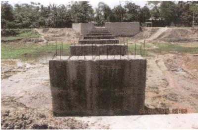
Aqueduct' on river Ghogra at Ch 9,180 of Branch Canal-7 (9 May 2013)
