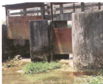
Main canal regulator at Ch 6,960 m (8 May 2013)
