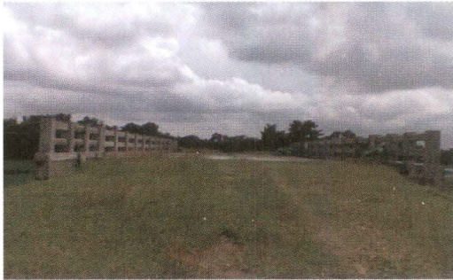
Bridge No. 30/2 on Dhubri Kachugaon Road (13 June 2013)
