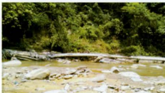
Broken channel at Fuanlui
