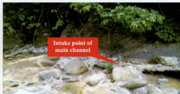
Channel without proper headwork at Fuanlui
