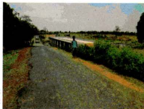
Bridge over river Bankal at 1 st km on Banki-Badamitalia road completed without construction of approach road
