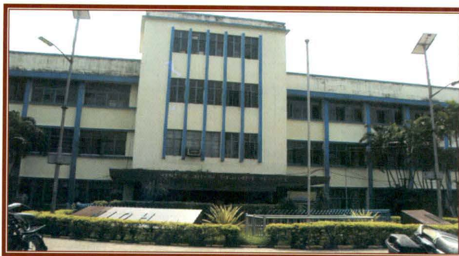
Front view of the NIOH building at B.T. Road, Bonhooghly, Kolkata
