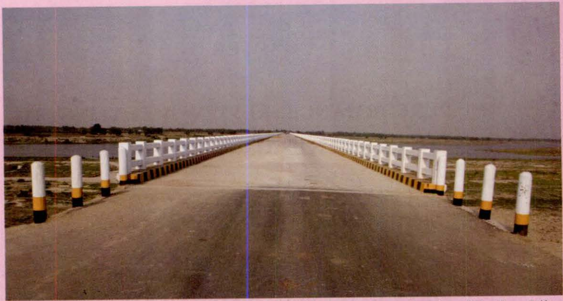
High Level Bridge Jhauo Across River Mahananda in the Dist of Katihar, Bihar
