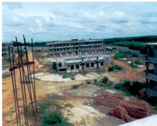
Central Prison at Bishalgarh scheduled in November 2009
