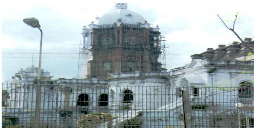
Seismic Retrofitting of Ujjayanta Palace scheduled in October 2008
