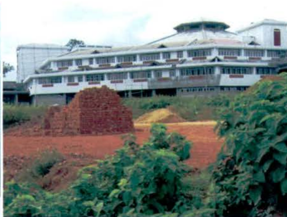
Construction of Assembly building scheduled in January 2009
