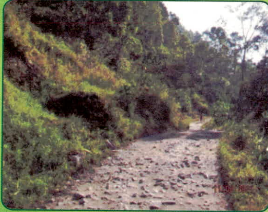
Narrowing of road due to landslide (8+ mile PWD road to Salghari JHS under Salghari GPU)
