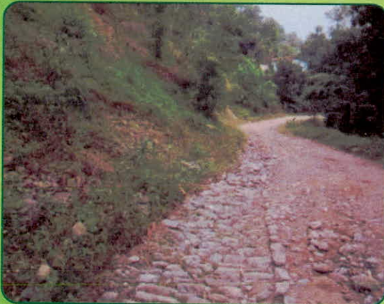
Narrowing of road due to landslide (Namphing Turning to Tshalamthang JHS under Namphing GPU)
