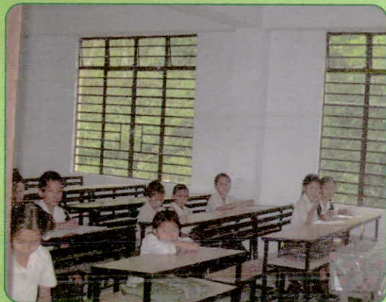
A good classroom of Lower Chalamthang PS under Namphing GPU
