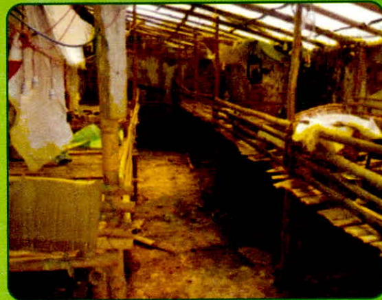
Empty poultry shed at Poklok-Denchung GPU
