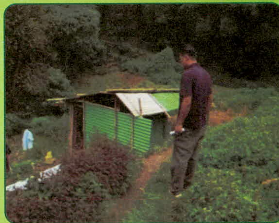
A shed constructed under RHS at Assangthang GPU
