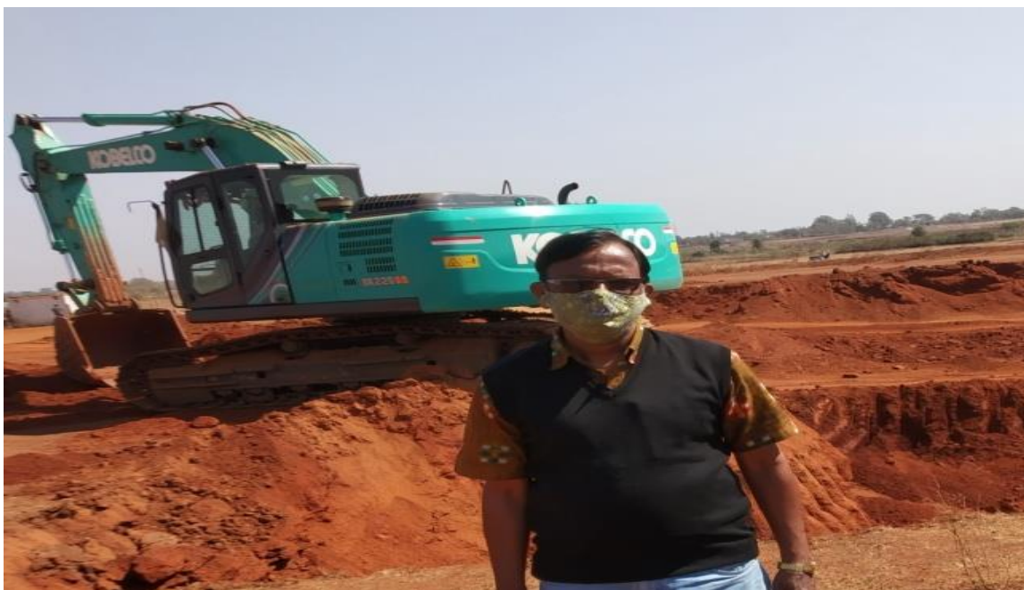
Figure- 4.5 (b): Murrum excavation sites (date of image: February 2021)
