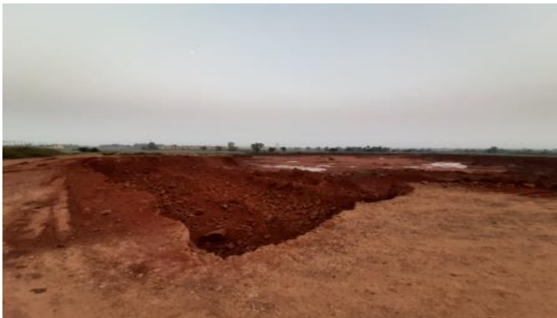
Figure-3.4 (b): Unauthorised murrum excavation near village Reco, Nava Raipur (date of image: October 2020).
