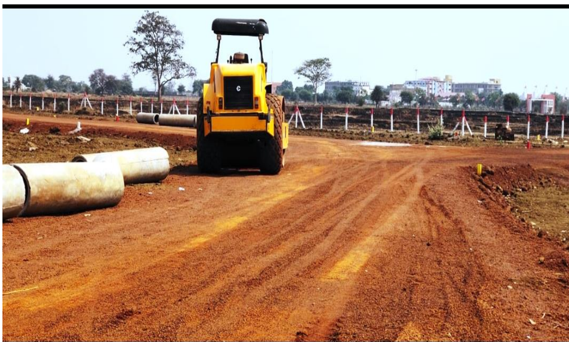
Figure-2.2 (a): Image showing usage of murrum at private construction sites (Residential Project, Raipur, month of image: September 2021)
