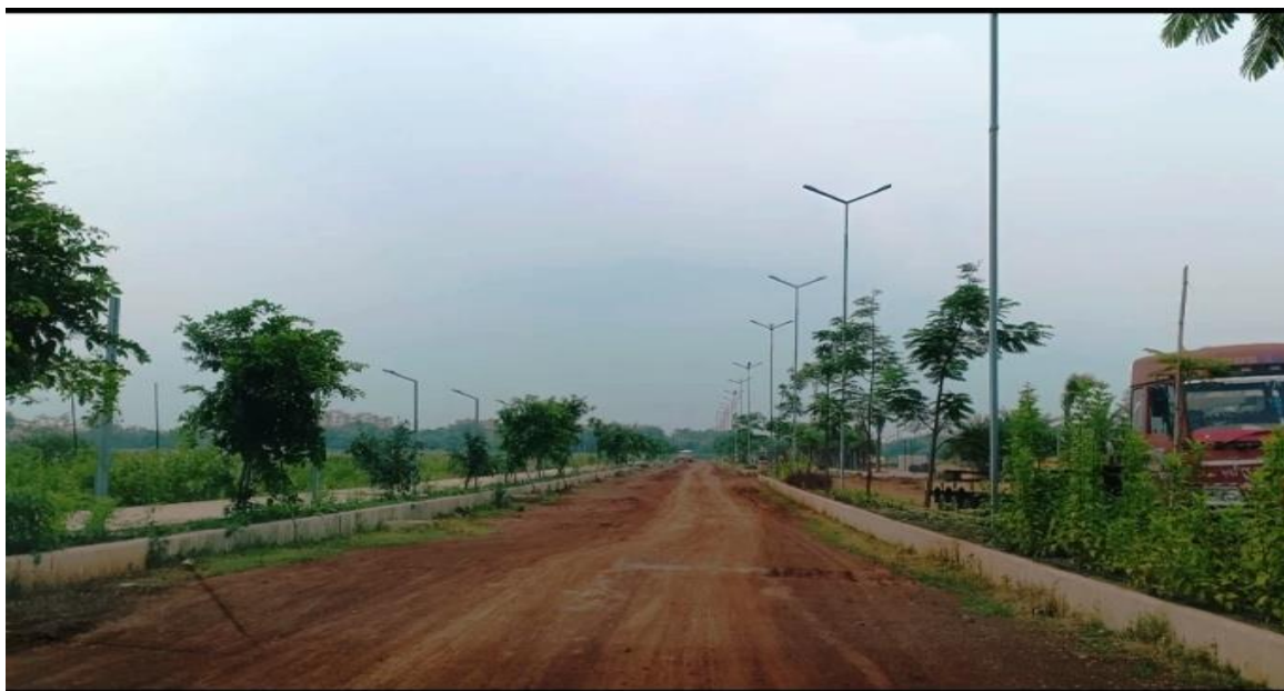
Figure-2.2 (b): Image showing usage of murrum at private construction sites (Commercial Project, Raipur, month of image: September 2021).
