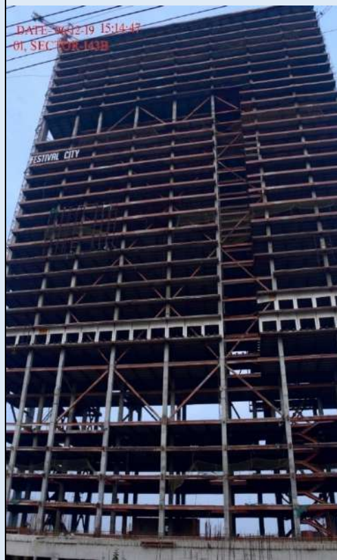
Photograph 5.3.2: Position of construction in December 2019
