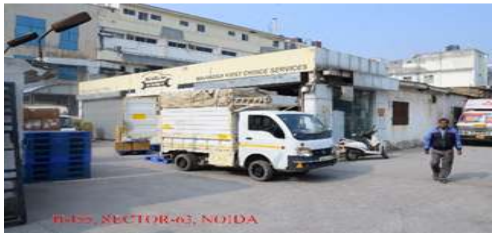
Plot No. H-155, Sector 63, Area 1,800 sqm Showroom of “Mahindra First Choice” being run on industrial plot
