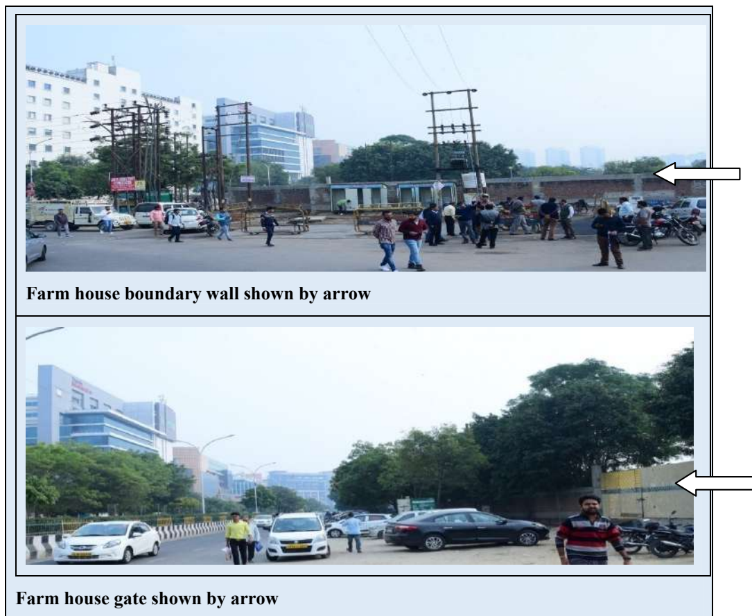
Photograph 5.3.7: Photograph showing physical location of farm houses in Sectors 126 and 127 opposite fully developed institutional plots
