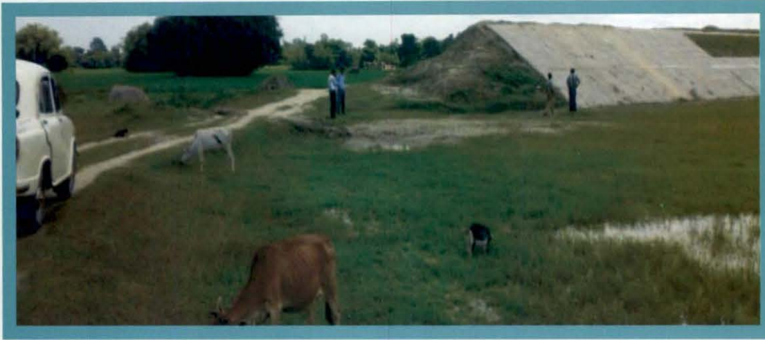
Teesta Barrage Project - West Bengal : DNMC of TBP at Ch. 63.585 where no trace of canal water was observed due to land dispute in Uttar Dinajpur District
