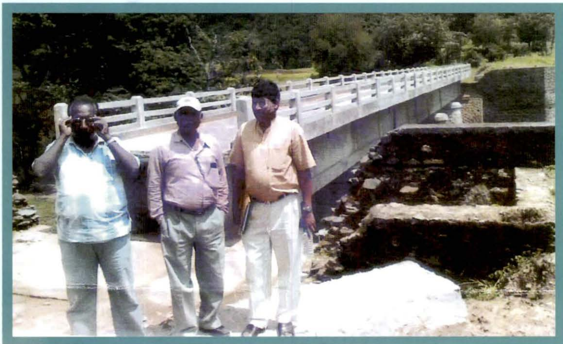
Incomplete aquaduct in Sonua Project
