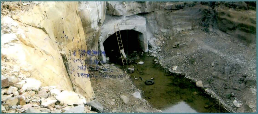
Incomplete Minors in Krishna Project
