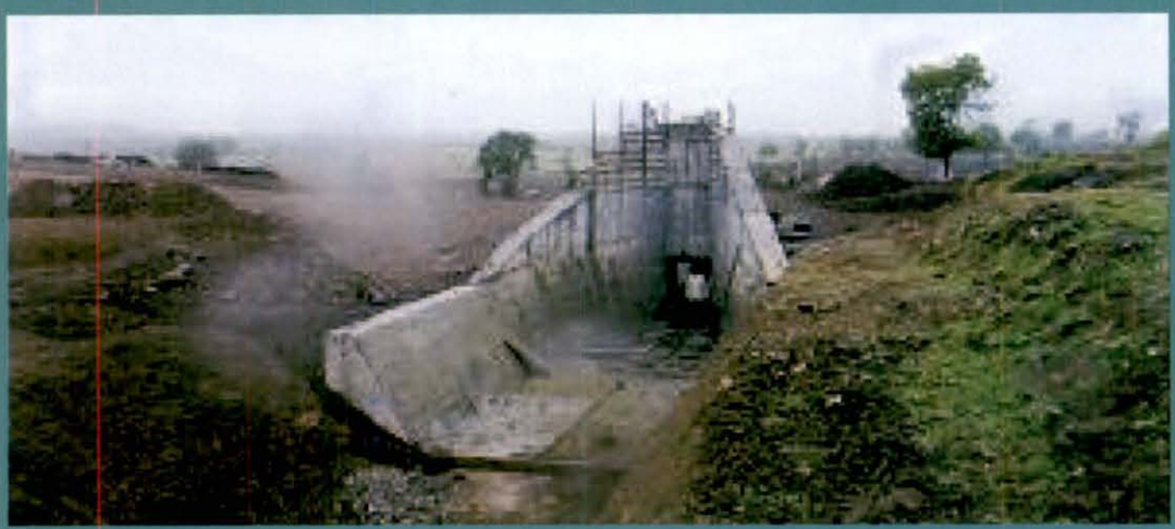
Canal work in progress in Kadakpurna River Project
