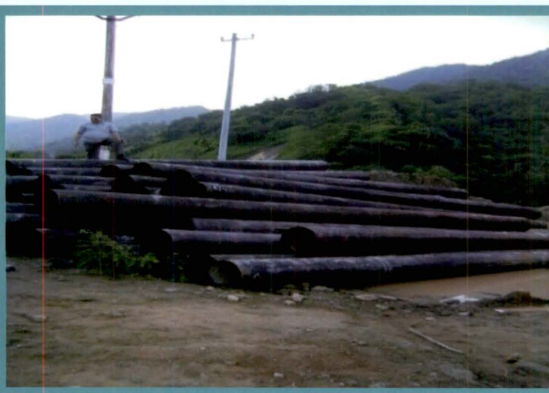
Non-laying of pipes of LIS Beh Maskar
