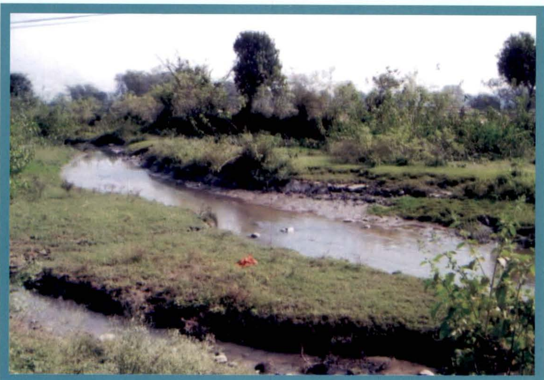
Unlined Portion of Basantpur Canal
