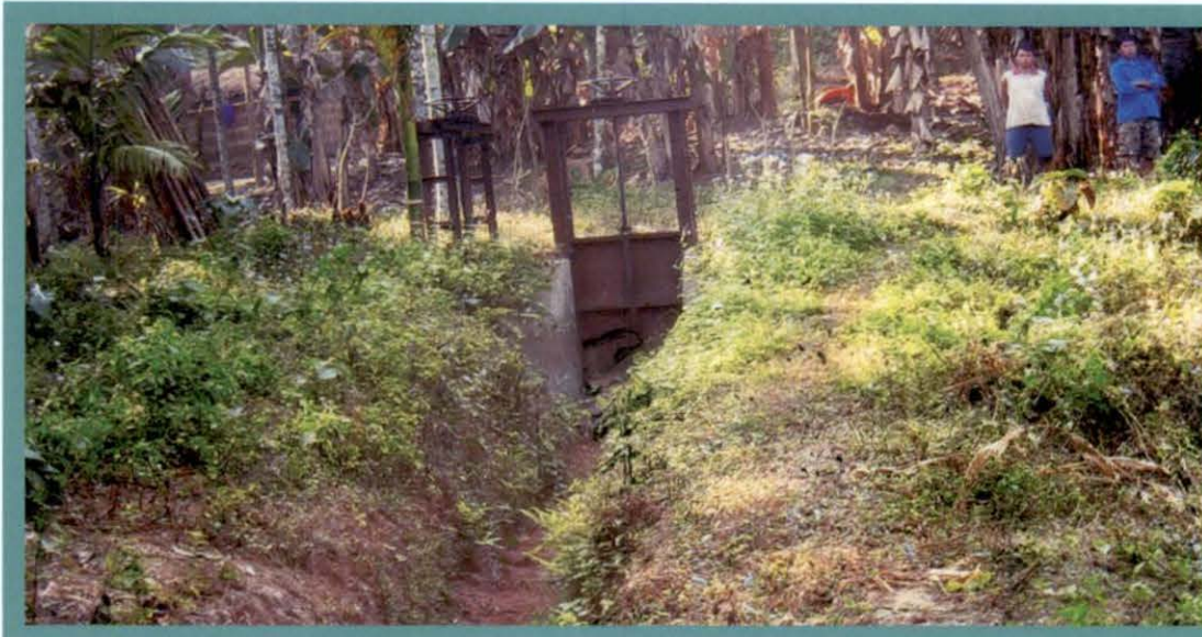
Gandual MI Project – Cross Regulator in the earthen canal with no water in the canal
