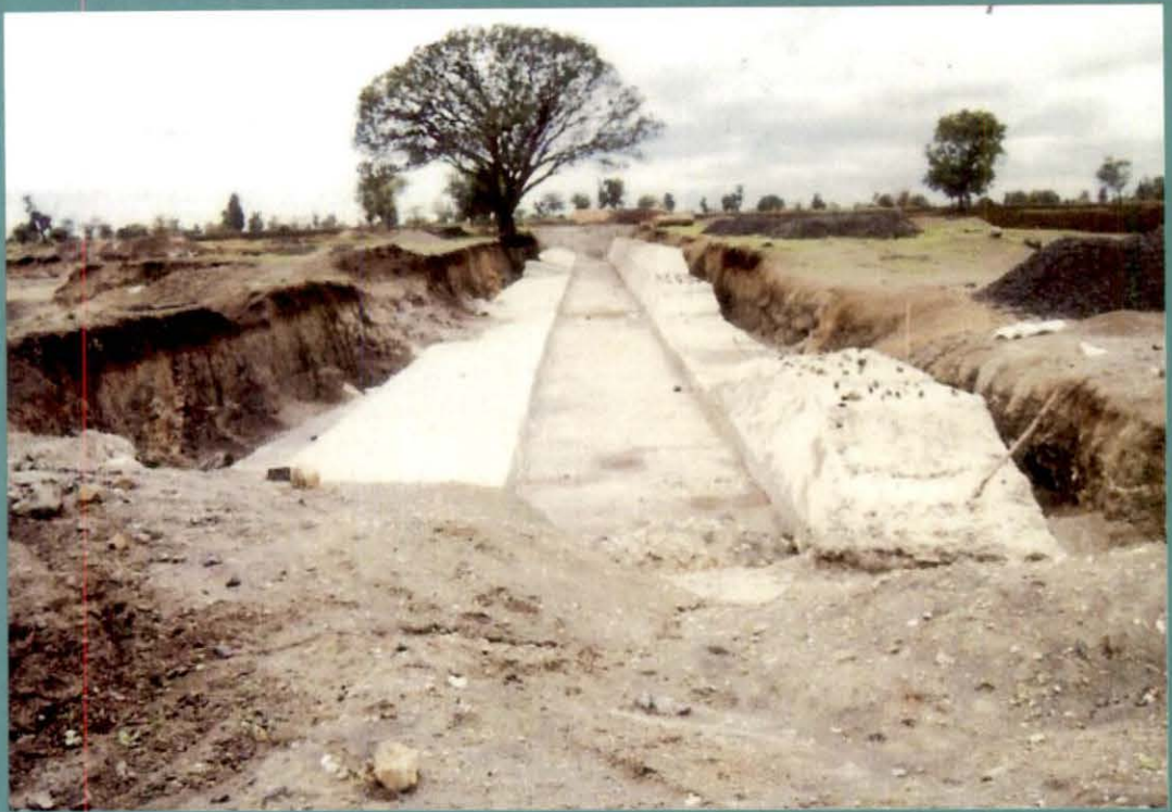
Mirzapur MI Project – Non-completion of canal work due to land acquisition problems
