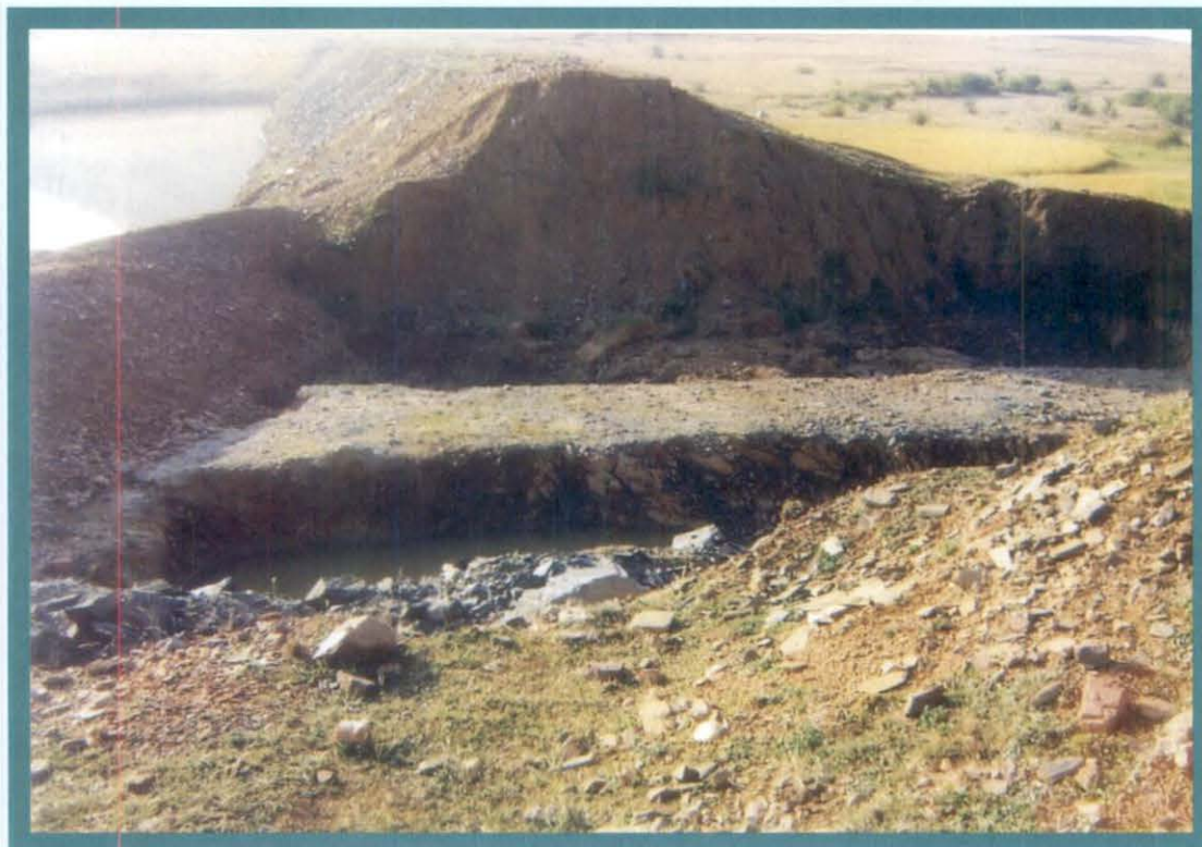
Incomplete spillway of Nayaki Reservoir Scheme
