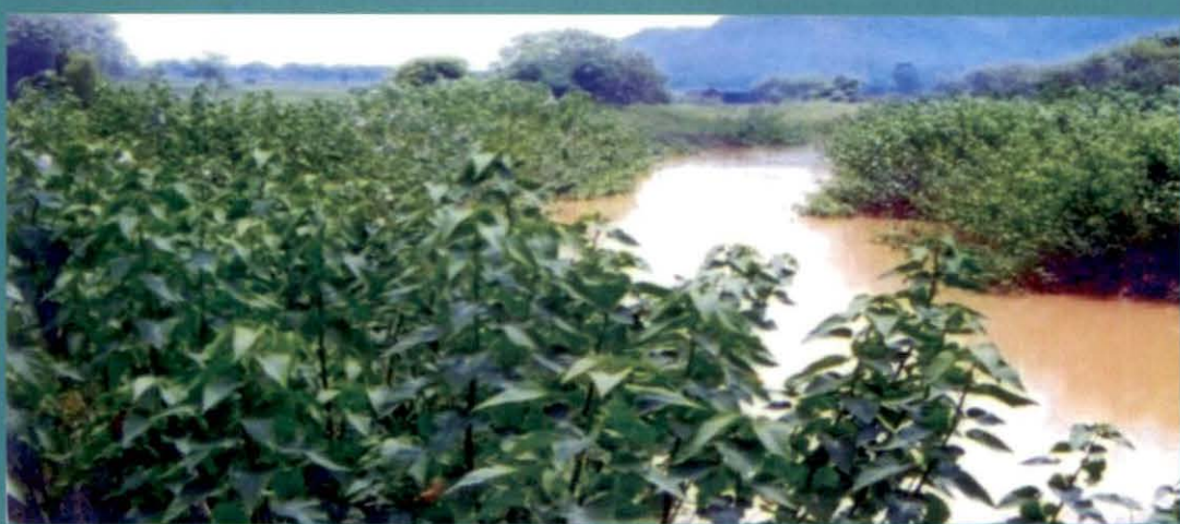
Sone Canal Modernisation Project (SCMP) - Bihar : High vegetation
