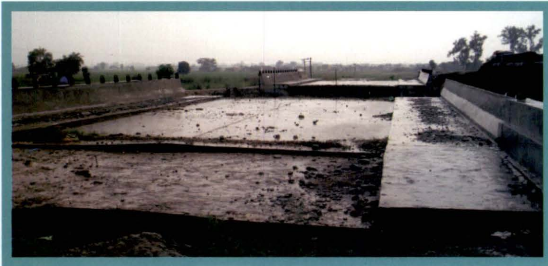
Agra Canal Project
