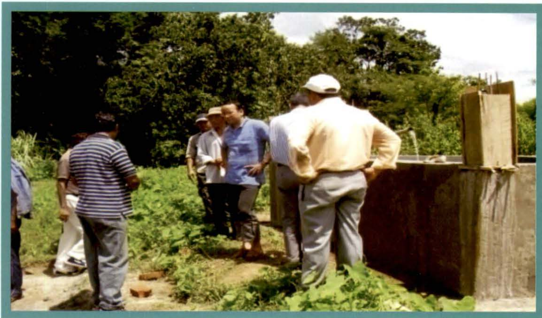
Reservoir under construction in Saihapui MI Project under Kolasib division
