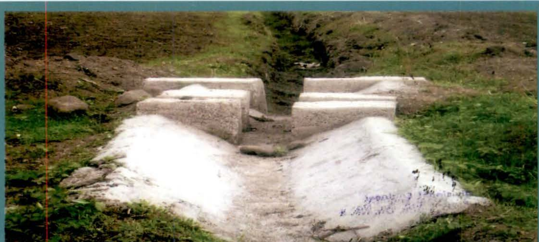
Slow progress of canal works in Arunawati River Project
