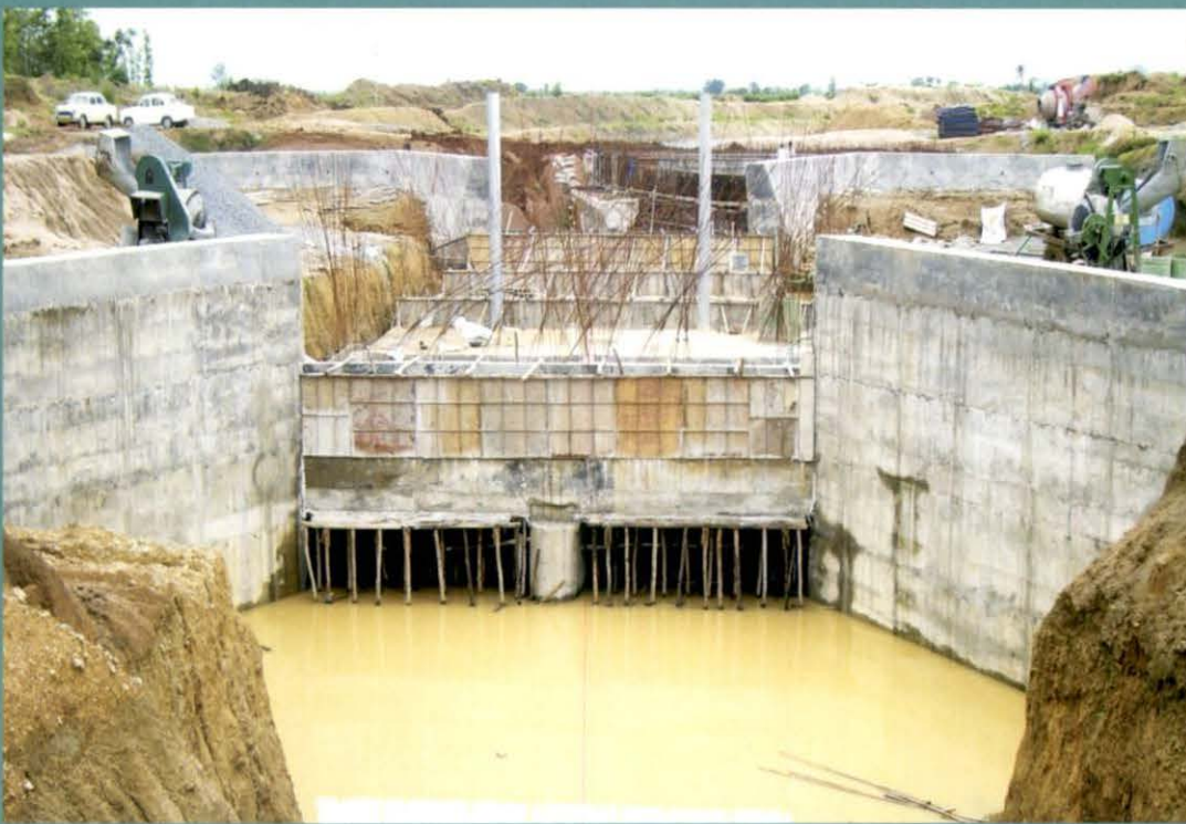
Ongoing work at Thotapally Barrage Project, Vizianagaram District
