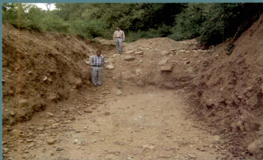
Pattra Cutting Work in Progress
