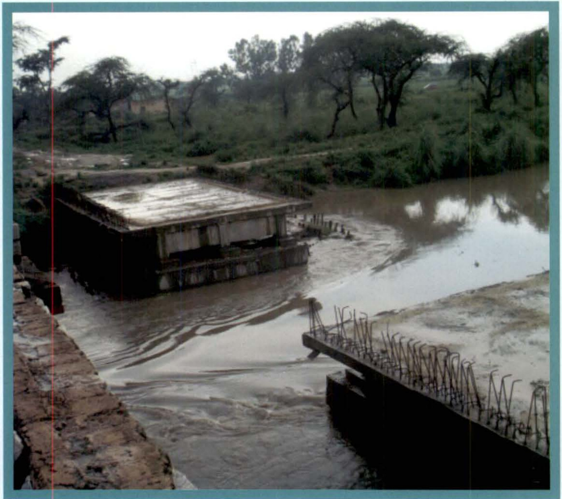
Agra canal project
