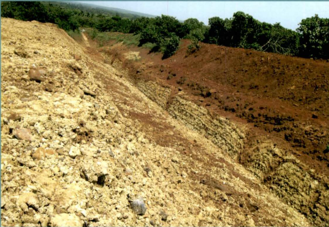
Ongoing canal work in Yerrakaluva Project, West Godavari District
