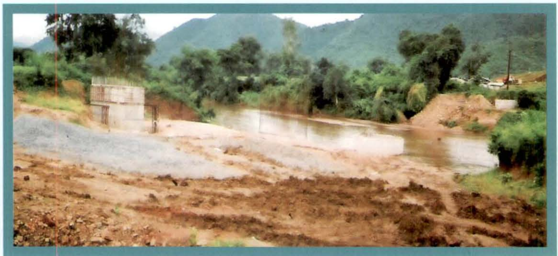
Upper Indravati Irrigation Project – Syphon Aquaduct over river Sagada at RD 2820 metre of REMC remained incomplete due to non finalization of design
