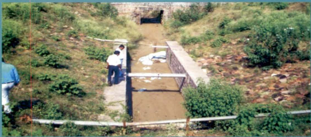
Rajghat Canal Project – Uttar Pradesh : Defective canal crossing at Km 0.750 of Bhailwara distributary below rail line and damaged canal due to back flow in the up stream of rail line
