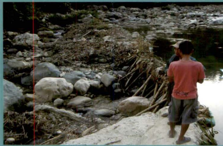
Damaged headwork and makeshift arrangements at Sille to Dekam MI Project at Ledum, Pasighat Division
