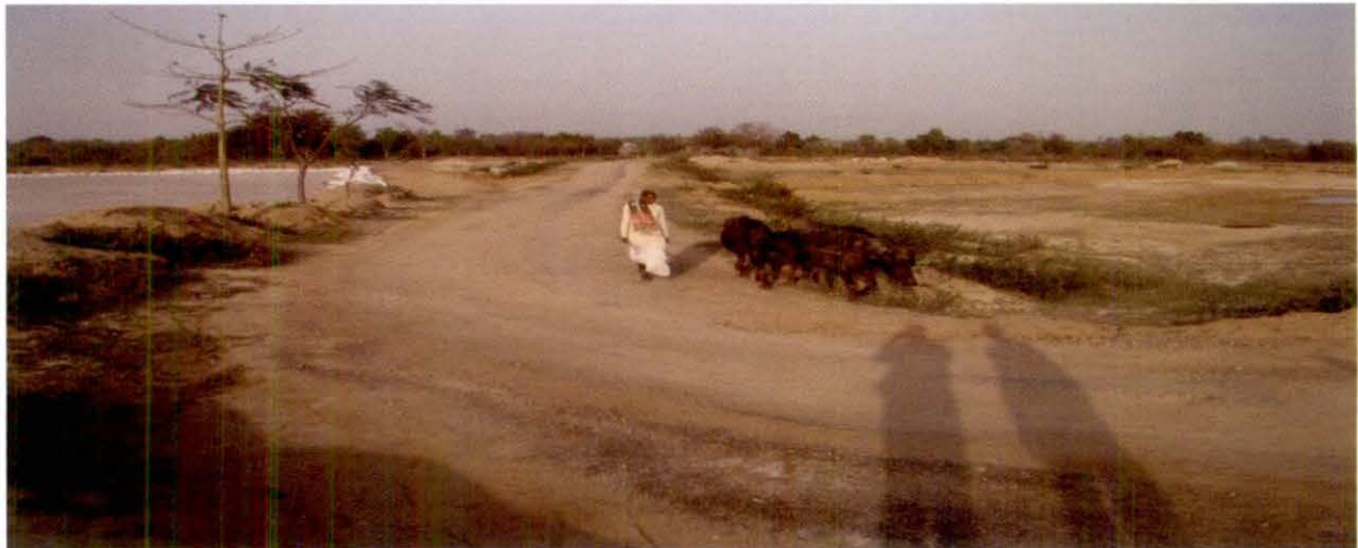
Picture 3: Road under Gramin Sadak Yojana of Rural Works Department, GoJ passing through ash pond area of KTPS
