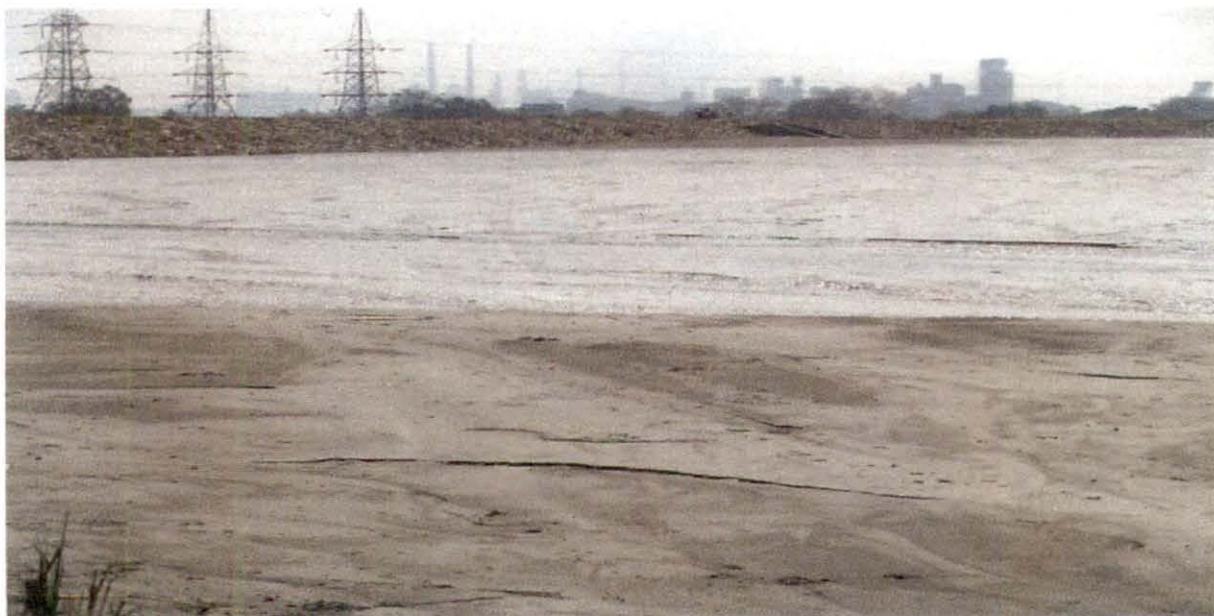
Picture 2: Filled up Lower capacity lagoon of Ash Pond – DSTPS
