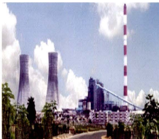
Picture: 1 Power plant
