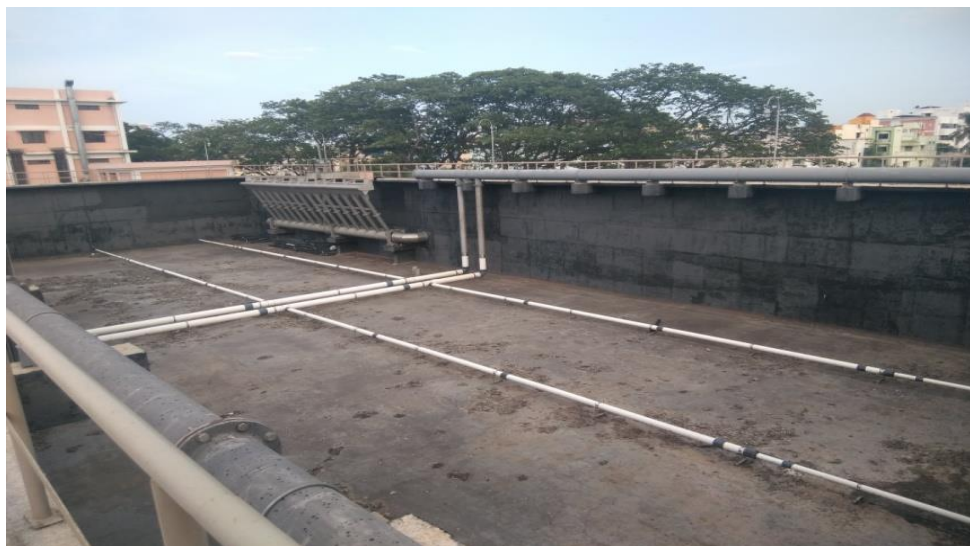
Picture 2 – STP under construction at Kanaganeri (5 July 2017)
