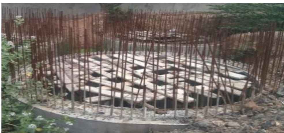
Picture 1 – Unfinished pumphouse at Kanaganeri (5 July 2017)
